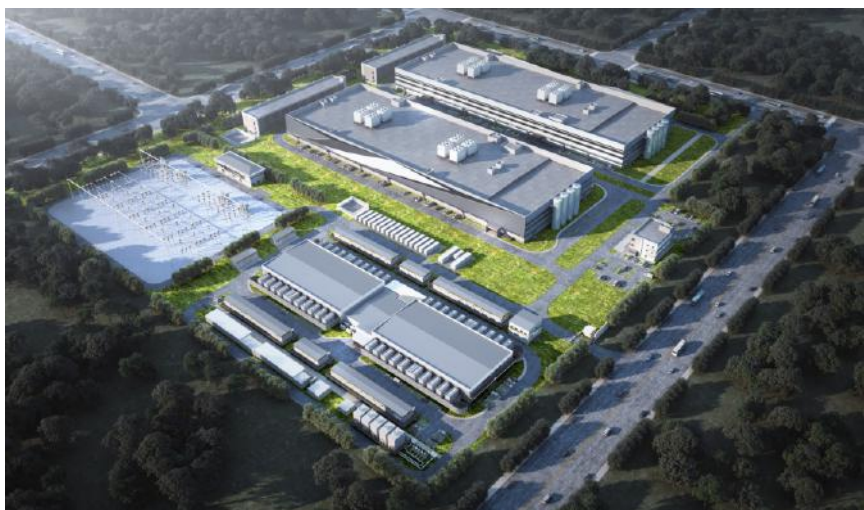
Aerial view of Chindata Group's data center in Malaysia
